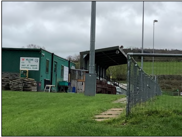
Plate 7: view of B2 and B3 onsite. Negligible potential for roosting bats.
