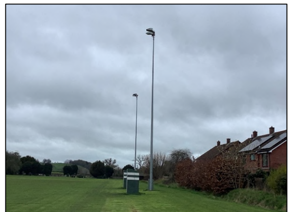
Plate 6: view of football pitch lighting offsite.
